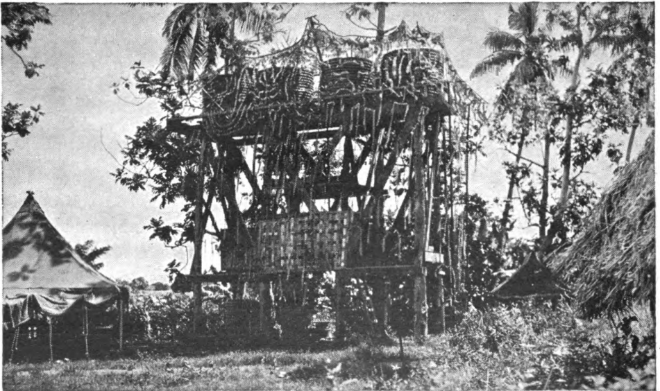
Figure 159. Elevated water tanks with chlorinating unit on intermediate stage.
